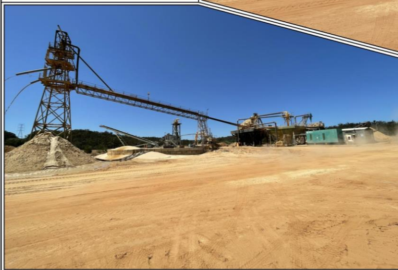
Plate 3: Sand loader and stockpile (Ref: E9801_039)
