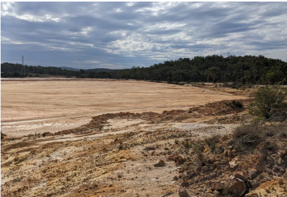
Photograph 3.2 A section of Domain 4 undergoing final profiling in preparation for revegetation
