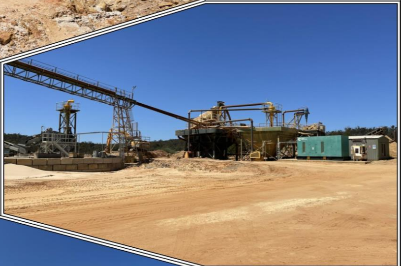
Plate 2: Sand loader and generator (Ref: E9801_038)
