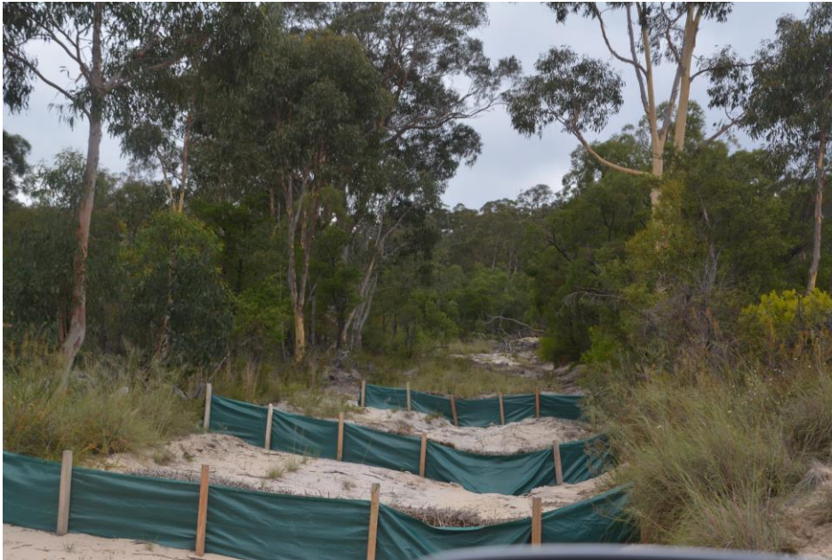
Plate 1 Hay bales and sediment fencing within the ephemeral drainage at the head of Tinda Creek (REF: E980A_065)
