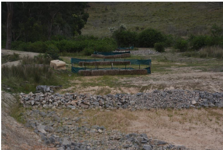
Plate 2 Sediment trap, hay bales and sediment fencing within a clean water diversion (REF: E980A_046)
