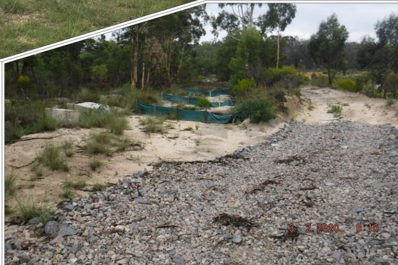
Plate 4: View of erosion sediment controls in the headwaters of Tinda Creek - February 2020 (Ref: E980B_007)
