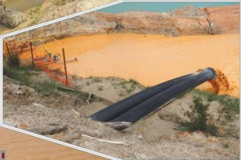
Plate 6: View of the New 300m Safety Overflow Pipes installed between the Sediment Pond and Dredge Pond - February 2021 (Ref: E980B_105)
