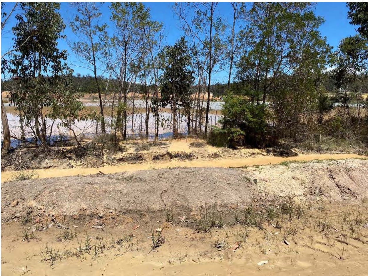
Figure 3. Overflow from Tinda Creek Quarry tailing pond, flowing upstream of Site 4.
