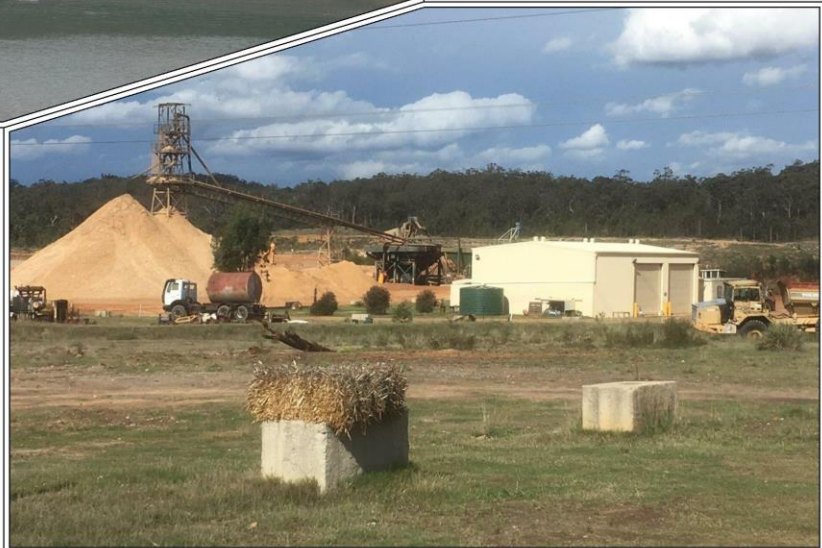
Plate 4: Sand Stockpile and Plant Infrastructure - November 2017
