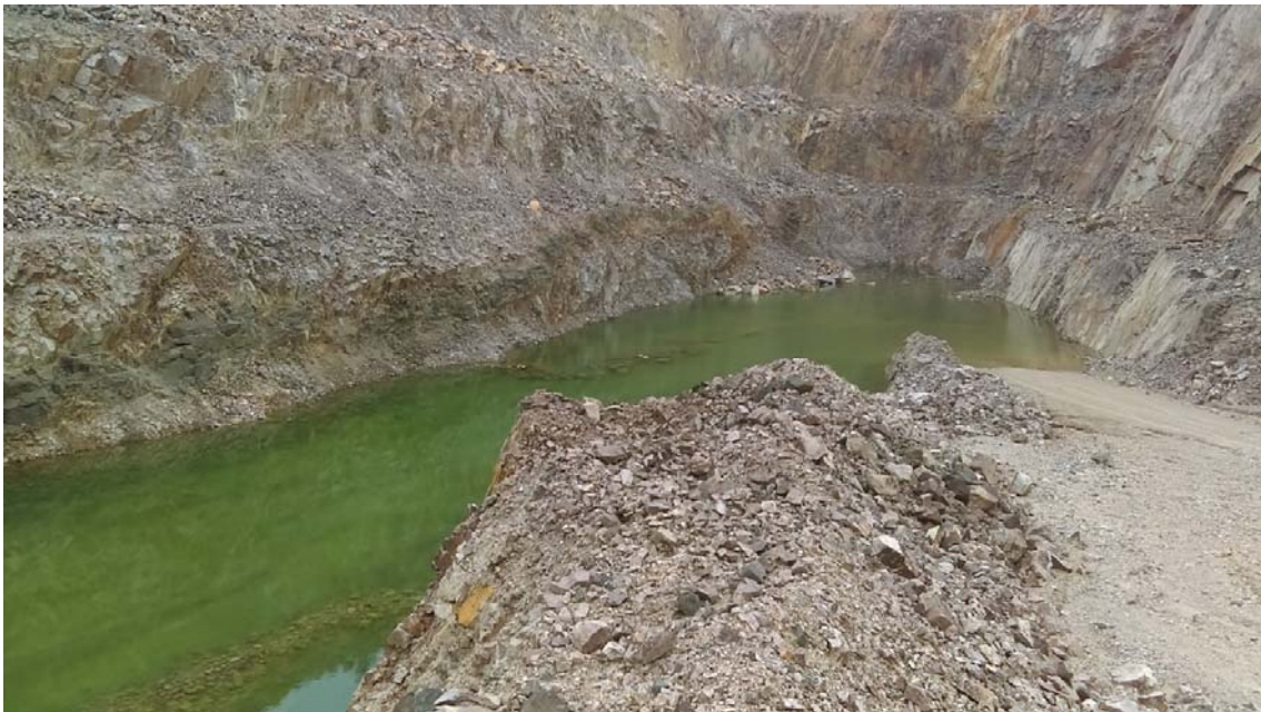
Photograph of pit from lower ramp. Photo taken at 0930am on 3 January 2019.
