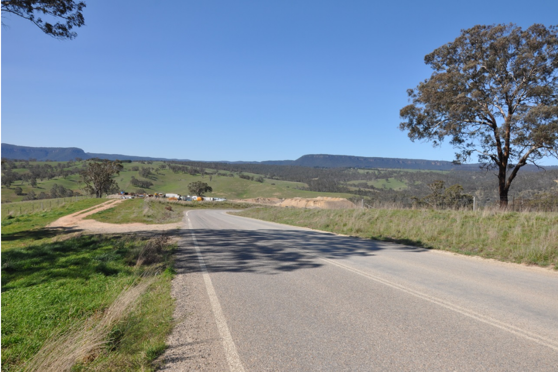
Plate 3.1: Section of Quarry Access Road West of Yorkeys Creek Stockpile Area
