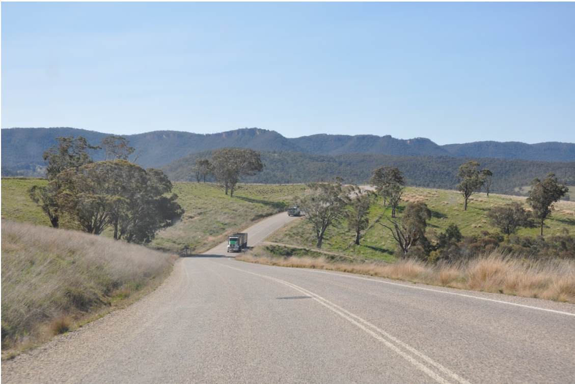
Plate 3.2: Section of Quarry Access Road Approaching the Quarry Entrance
