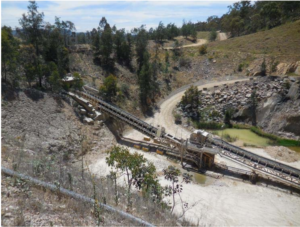
Photograph 7: Conveyors from primary crusher.
