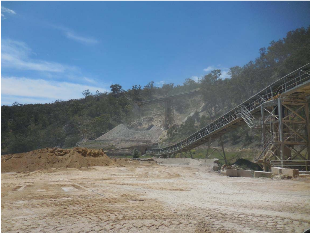
Photograph 3: Raw material stockpile and conveyor. Dusty conditions around the end of the raw material conveyor and in the processing area were noted.
