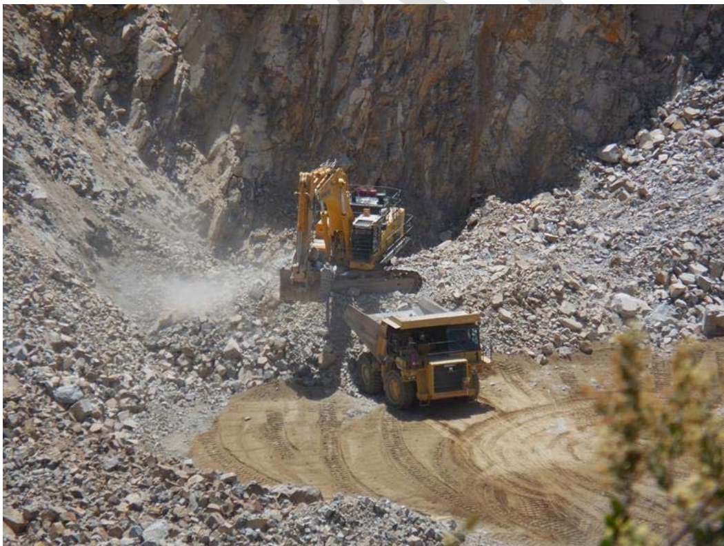
Photograph 8: Excavation of material in pit.
