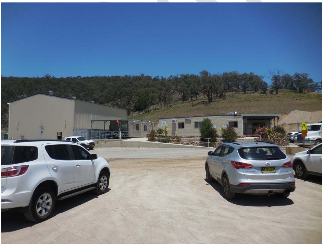
Photograph 4: Offices and car park.
