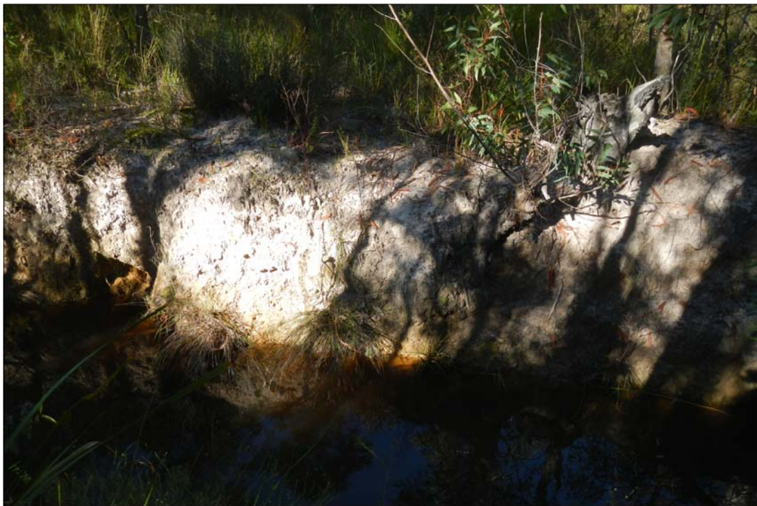
PLATE 30 View of excavated drainage line at 286463 6328666 showing soil profile (loose sands).
