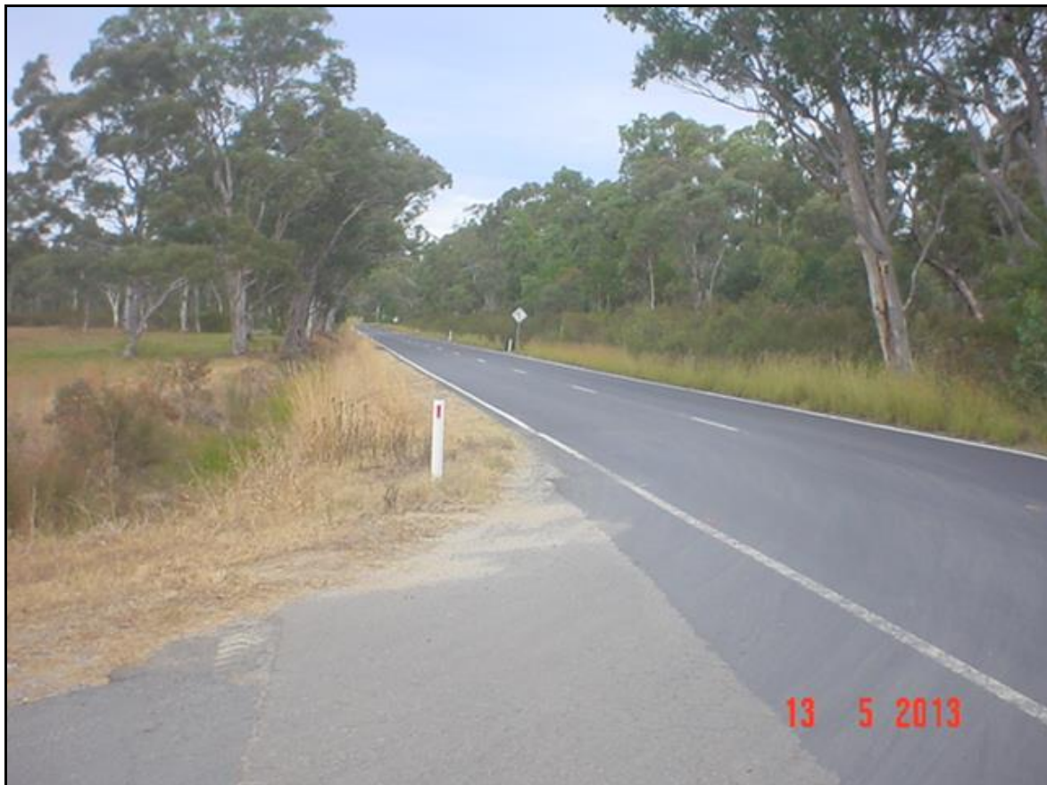
P1 – LOOKING SOUTH ALONG PUTTY ROAD FROM QUARRY ACCESS
