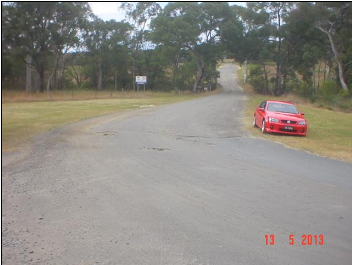
P3 – QUARRY ACCESS ROAD APPROACHING PUTTY ROAD
