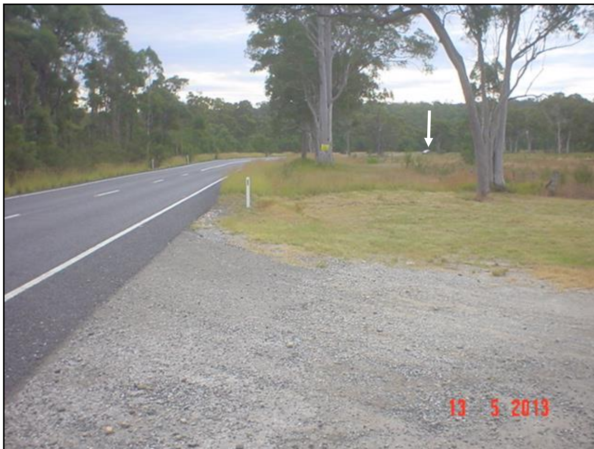
P2 – LOOKING NORTH ALONG PUTTY ROAD FROM QUARRY ACCESS
