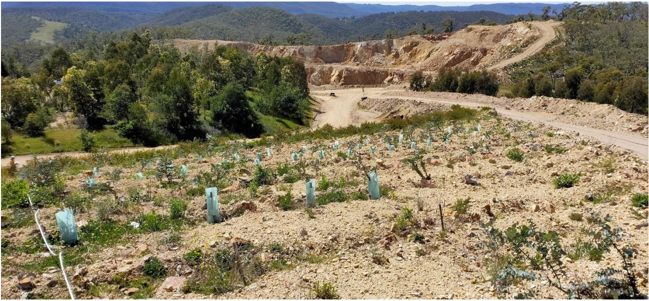
Photograph 4.8 View across New Rehab site looking East
