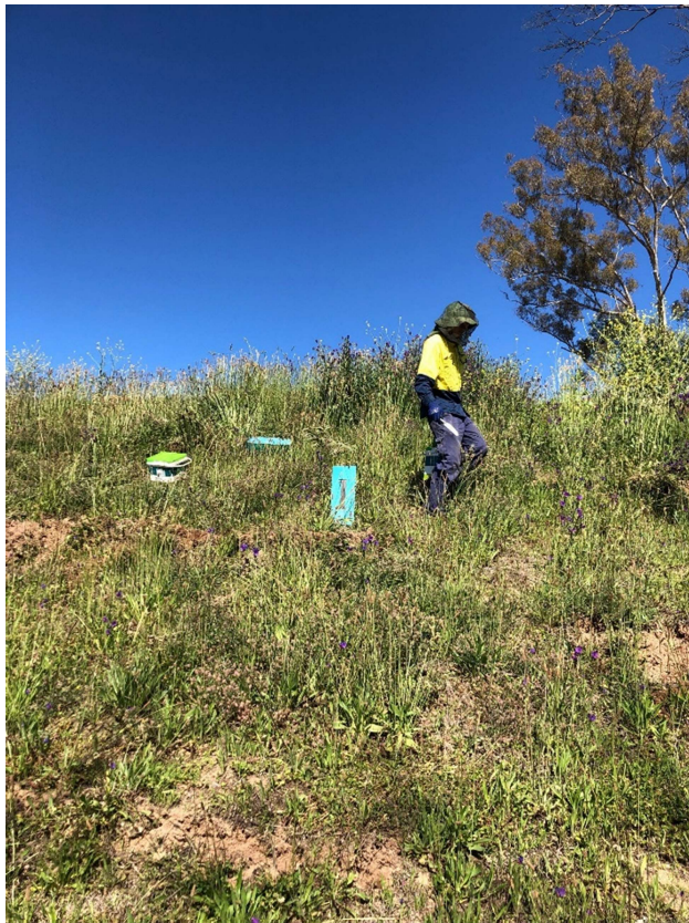
Land Works crew installing plants at Western Boundary site.
