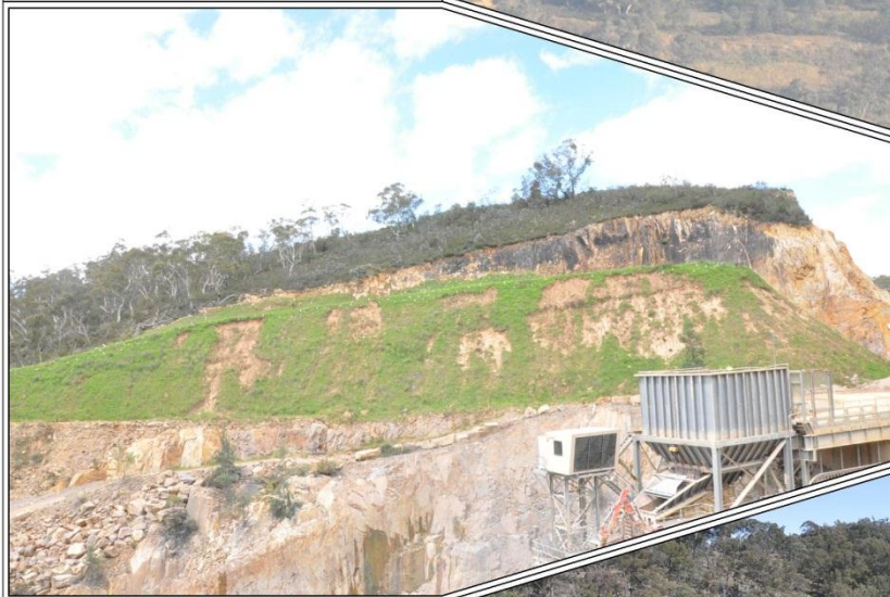
Plate 4.3: Established grass coverage of Northern Extraction Face (Ref: E652S_027)
