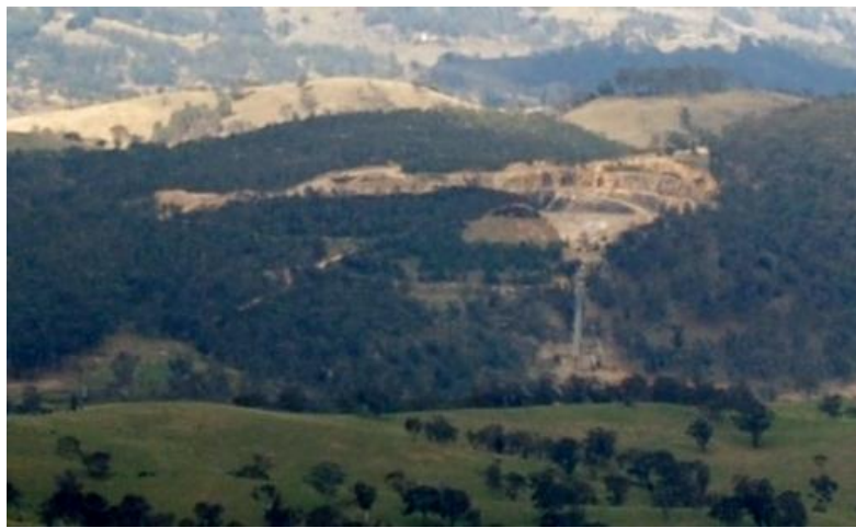
Plate 1.9 Extraction Face pre-Bituminous Film re-application (20/9/2013)
